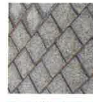
Trafficable pavement sets
